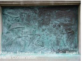
the future by cleaning and application of a protective wax coating this finish may be considered as contributing to the visual appearance of the memorial. However, if the corrosion is active as discussed above, then it will need to be removed to protect the bronze.
