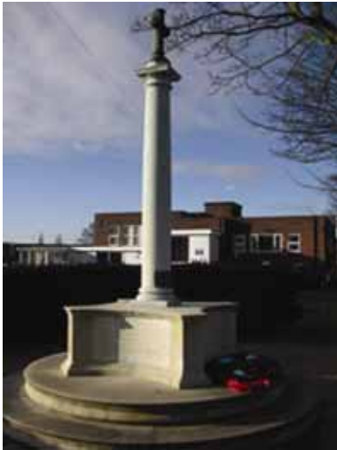
After work completed © Bestwood St Albans Parish Council, 2008
