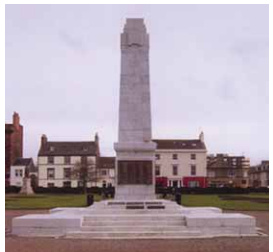
After work completed © South Ayrshire Council, 2008
