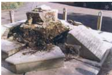
The foundations © Burlite Ltd, 2008
