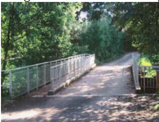
Bradshaw memorial bridge
