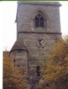
Shireoaks clock tower
