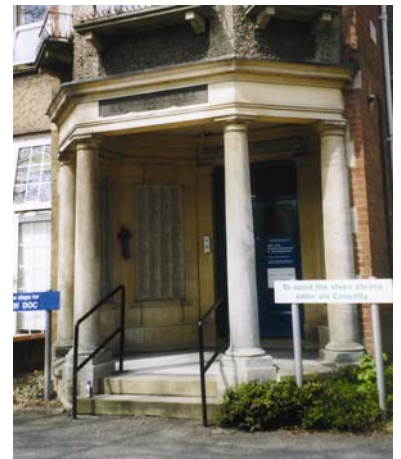
Hospital portico © D. Kenyon, 2008
