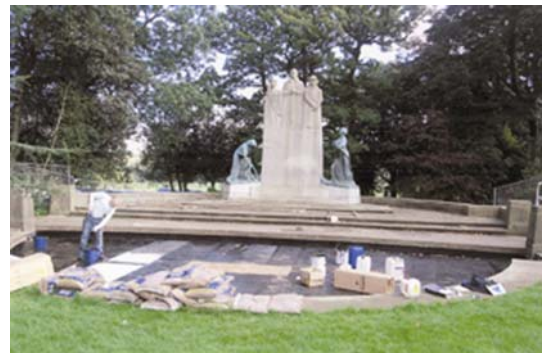
During works to the pool © Burnley Borough Council, 2009
