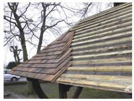
Replacing the roof shingles onto timber battens © Kennington Community Forum, 2010
