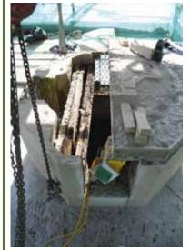
During works showing the heavily eroded metal supports inside the pedestal of the memorial © A. Williams, 2013
