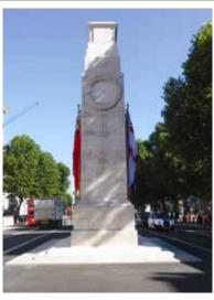
The Cenotaph following the cleaning and re-pointing work. Note in particular the difference in colour at the top of the memorial compared to previous images
