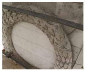
The extent of the staining can be seen when exposed areas are compared to sheltered areas, as seen on this wreath before cleaning
