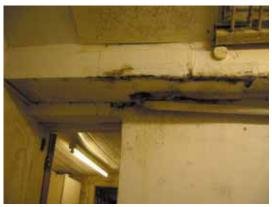
Internal damage by leaking roof © D Smith, 2013
