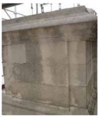
The top of the Cenotaph has the most severe staining
