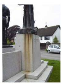
Staining caused by ferrous fixings within the structure © Cardiff Council, 2013
