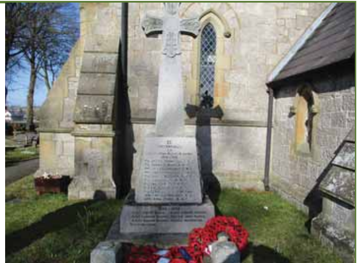
Brynford before (above) and after works (below left) (WM10126) © Brynford Community Council, 2021
